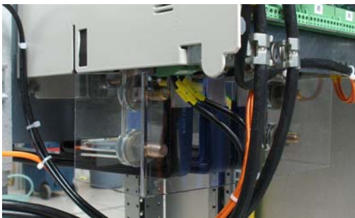
Examples for DC main terminal covers for D3 (left) and D4 (right) converter modules.
